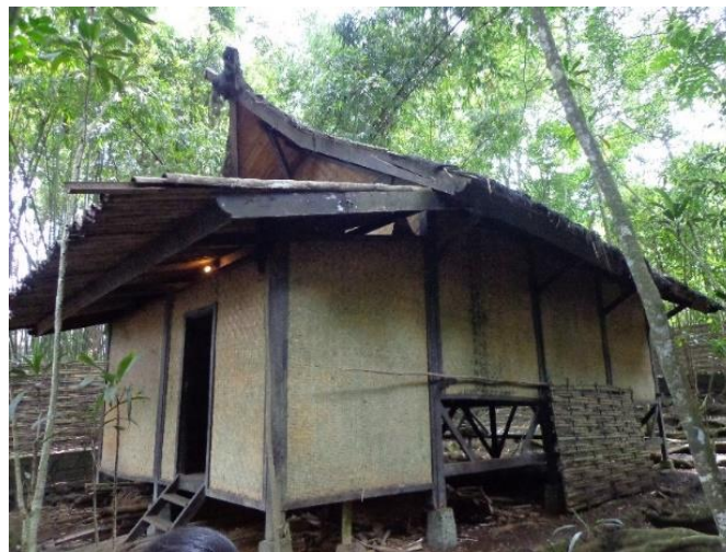
Figure 5: Padaleman building is a place to store Old Sundanese manuscripts in Kabuyutan Ciburuy. (Photo by the author)
